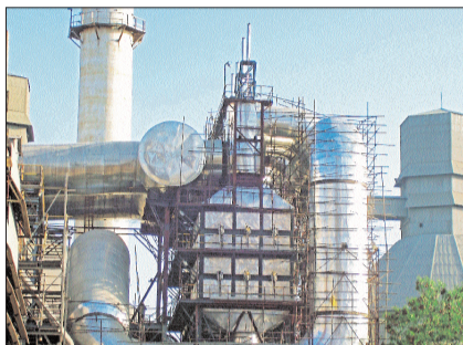
Waste Heat Recovery Thermic Fluid Heater in Cement Plant
