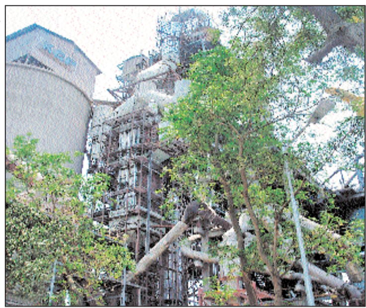
Waste Heat Recovery Boiler - Cement Plant
